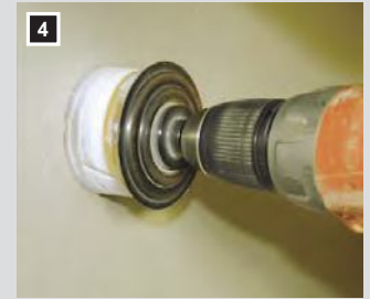
4 You can now cut-out the hole without remeasuring the installation site.
