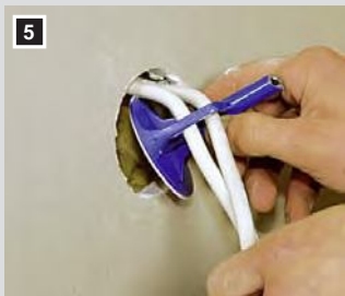
5 Pull bus holder and cables out of the wall.
