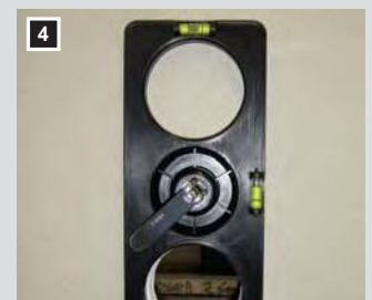
4 Fixing the drilling template with the spanner.
