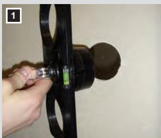
1 Drilling of central hole
