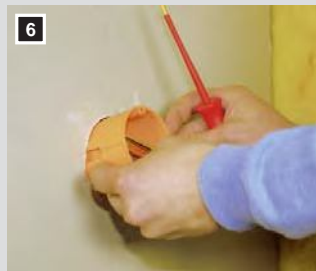
6 Install the cavity wall box without laborious searching for cables in the wall.
