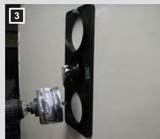
3 Thereafter, drill through the existing hole inserts.
